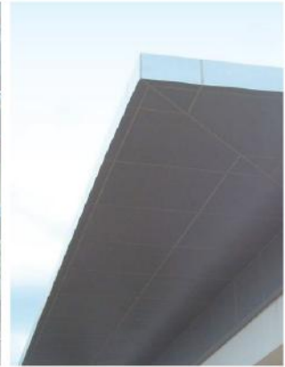
BuNos Fascias and Soffits
