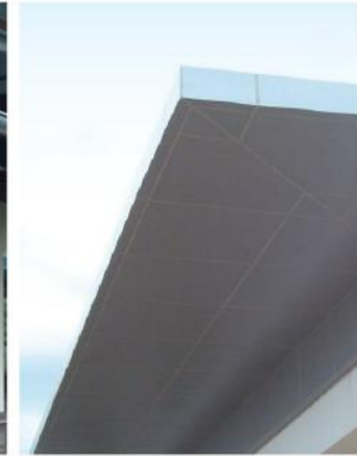
BuNos Fascias and Soffits
