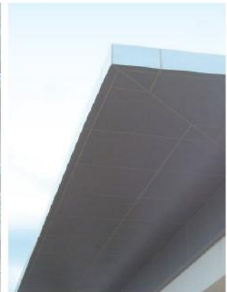
BuNos Fascias and Soffits
