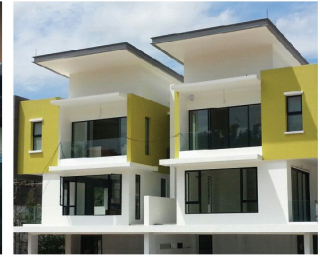
BuNos Fascias and Soffits
